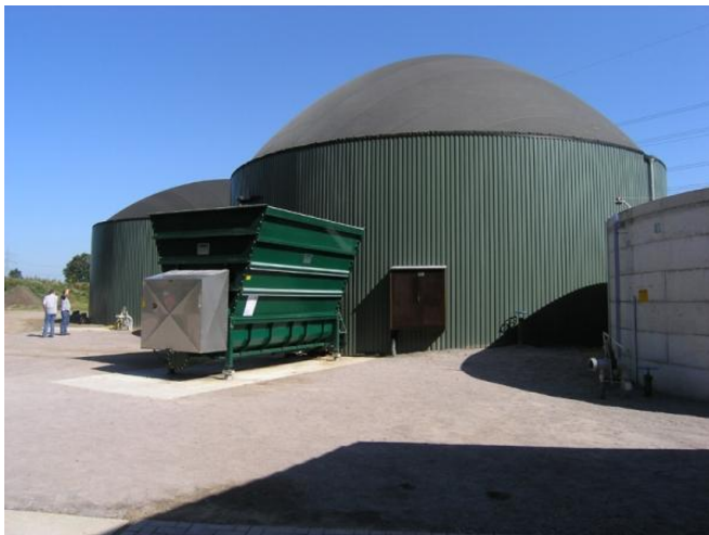
Figure 1 - Sample anaerobic digester
